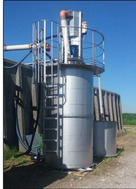
Microfiltration Test Farm 2
